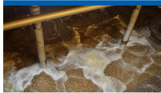
CFIC® reactor contains highly packed biofilm carriers to a degree (typically 90-99% bulk volumetric fill) that little movement of the carriers occurs in the reactor during normal operation.
