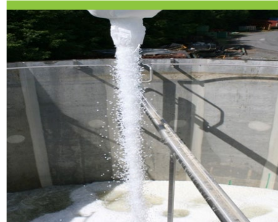
Bioreactor being filled with media.
