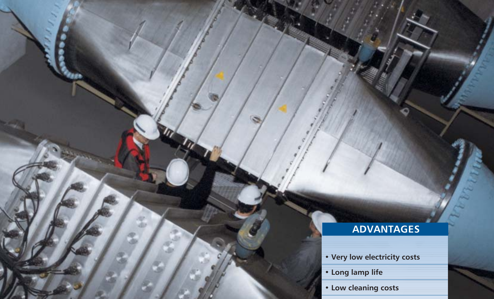
WEDECO UV disinfection system for Clayton County, Georgia, USA
