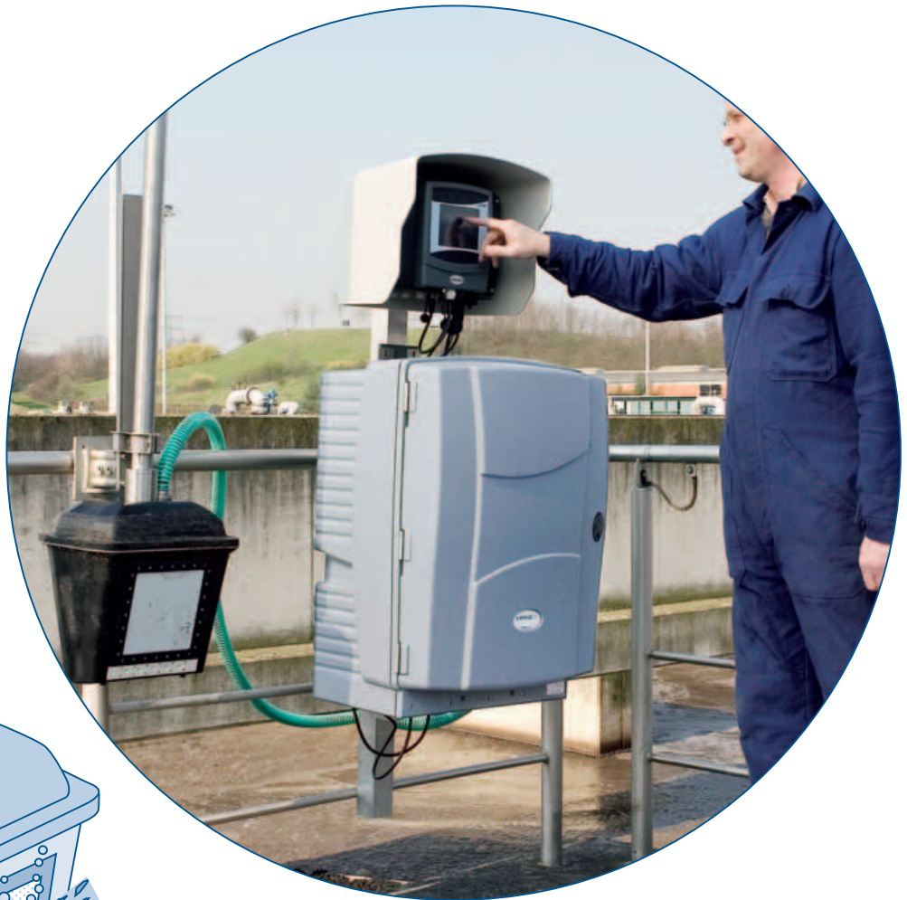
Filter probe in service position: the complete system is installed tank-side and requires very little space
