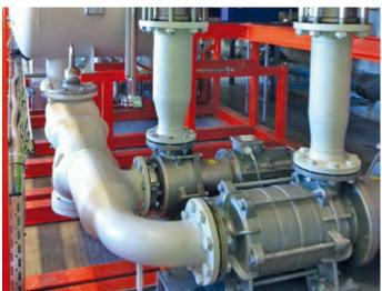
Furthermore these pumps are characterized by a compact design, open impellers without axial thrust or closed balanced impellers as well as diffuser devices in the circular casing that do compensate most of the radial forces. This among others has a positive influence on the magnetic coupling service life.
