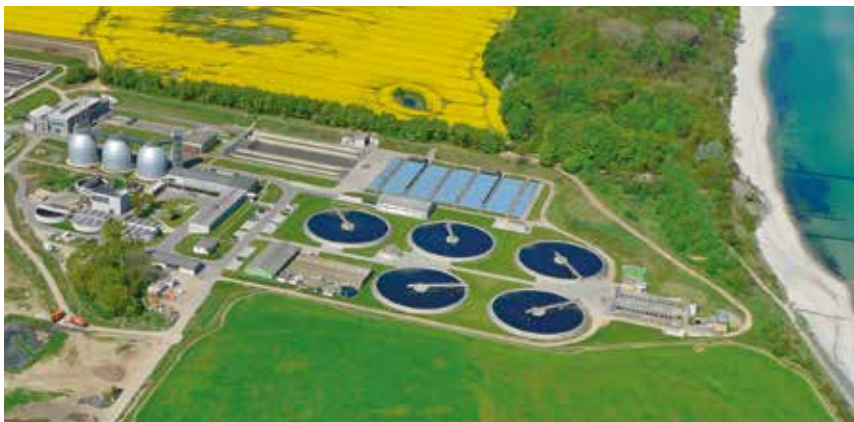
EDUR multiphase pumps successfully in operation at the municipal WWTP Kiel.
